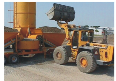
Plant working on Road project for Fly over construction
